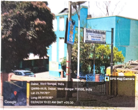
PHOTO-4 :- OFFICE OF ECL
